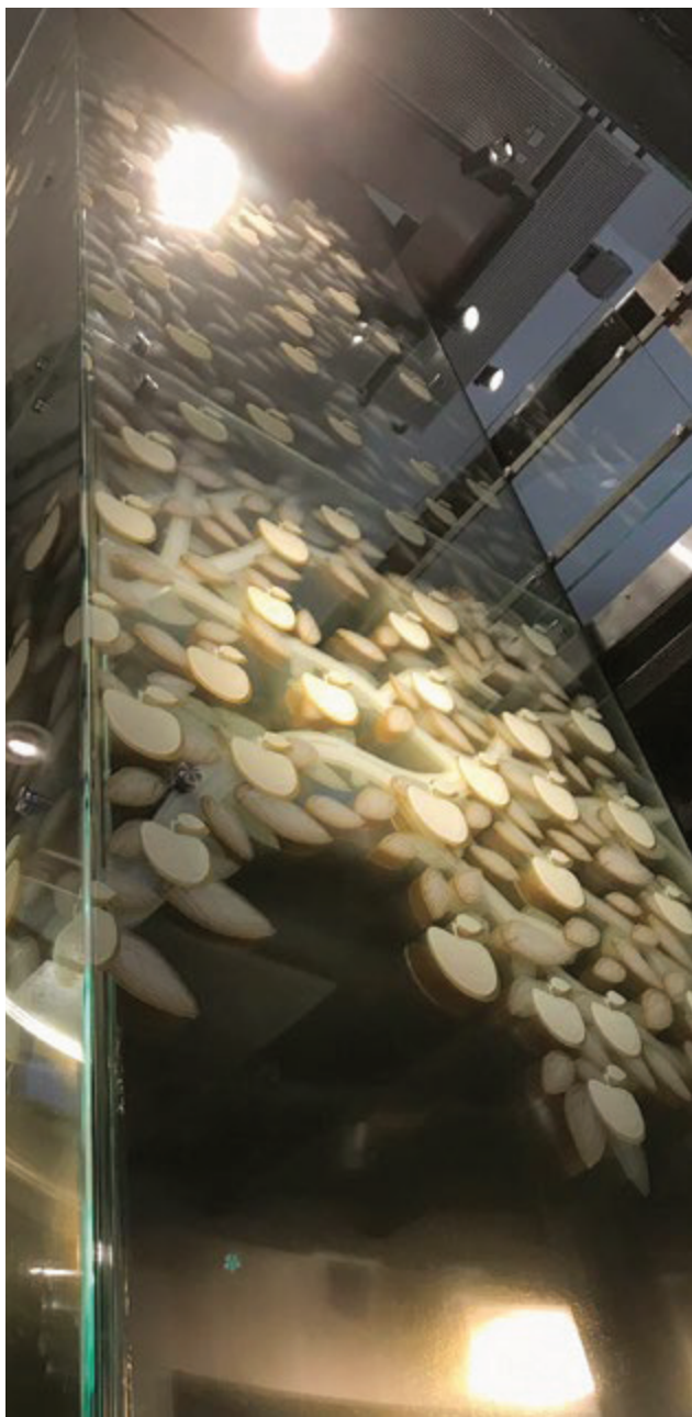
Artistic glass elevator finishing “Golden apple tree”, Knowledge center of Latvijas Banka “Money World”. Riga, Latvia Unique, artful, 10-layers glass construction, covered with gold. H 8m Architect: Agris Padelis-Lins, “Arhitekts Agris Padelis-Lins” IK Glass production and installation: “AM studio” LTD
